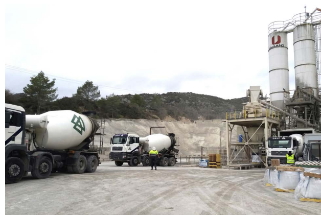
The Vallarca concrete plant (Barcelona) .
