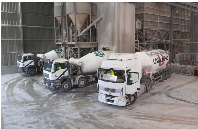
The concrete plant in the Free Trade Zone (Barcelona) .
