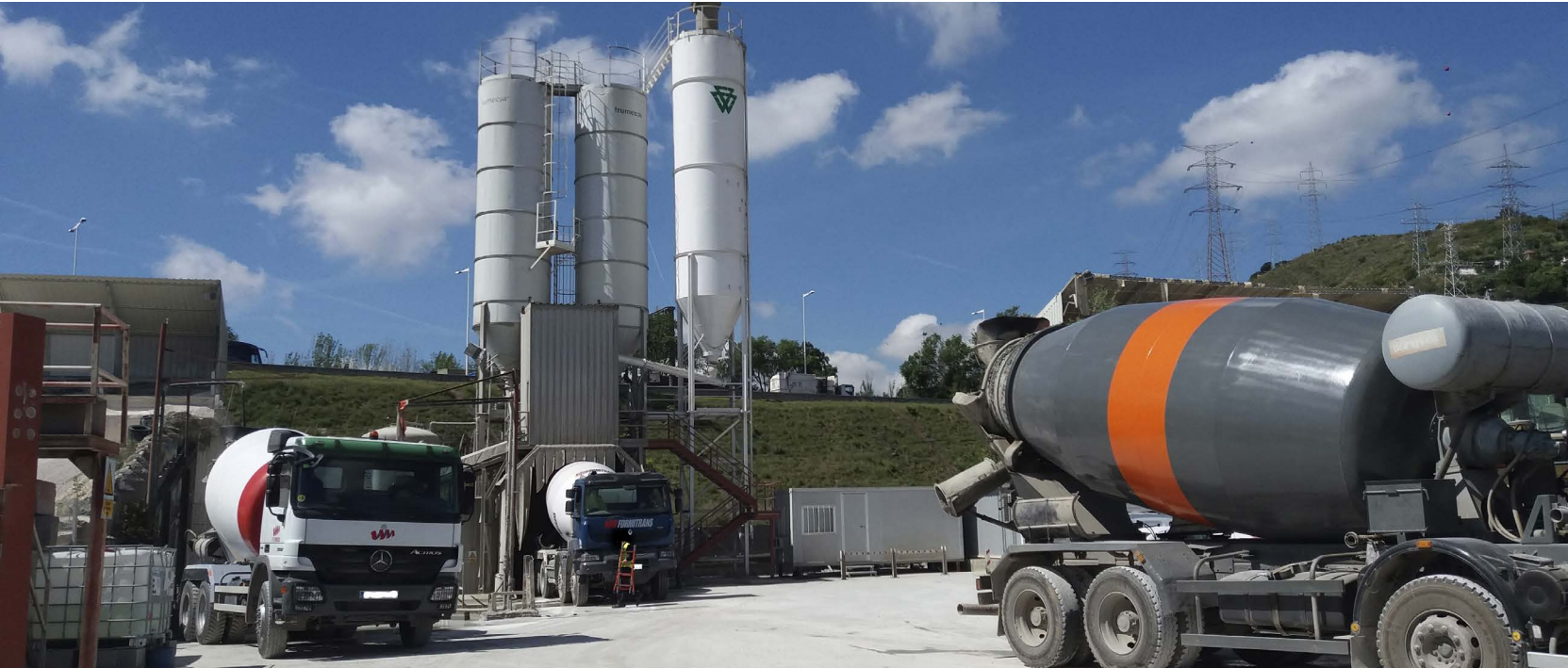
The Trinitat concrete plant (Barcelona) .
