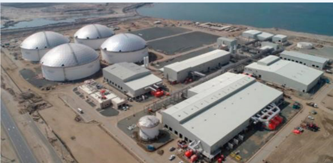
Aerial photo of Jizan industrial complex (Saudi Arabia).
