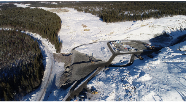
FCC Construcción won its first project in Norway with the award of the E6 Ulsberg-Vindasliene highway.
